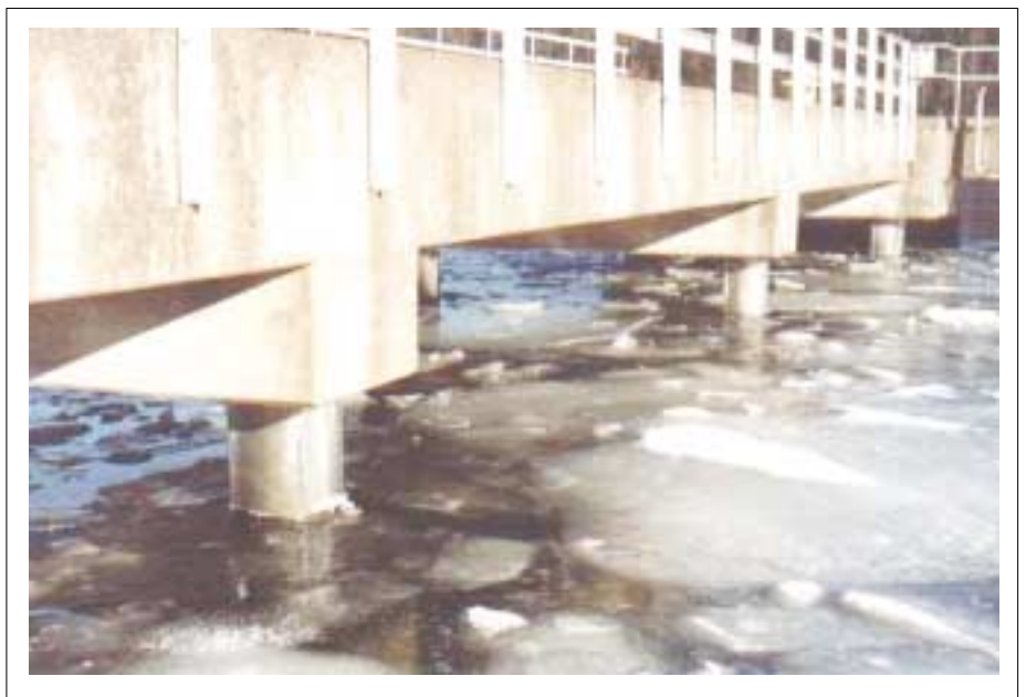
The oilharbour at Södertälje after tubular piling restoration
